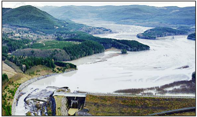
The sediment retention structure and upstream sediment plain on the North Fork Toutle River, flowing out of Spirit Lake. U.S. Army Corps of Engineers
